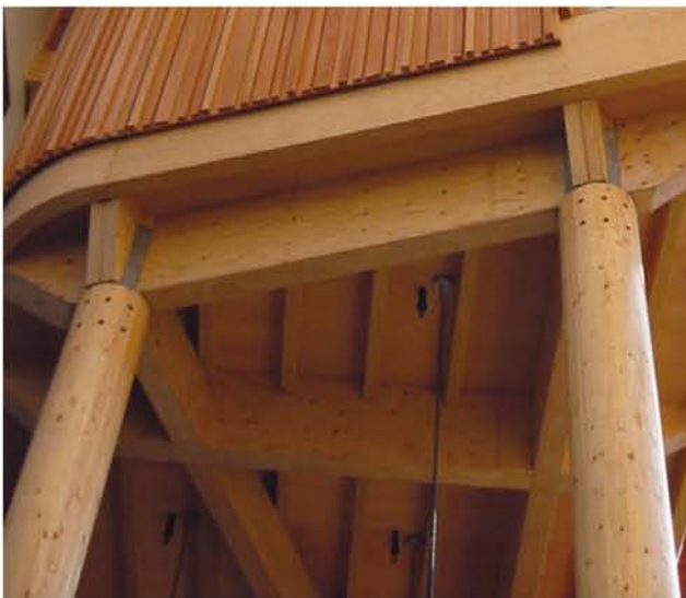
Glulam columns, LVL transoms
