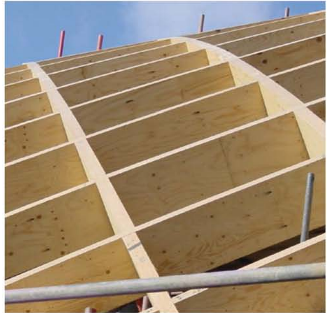
Laminated Veneer Lumber lamella roof
